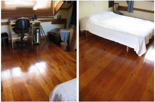
Figures: 27 and 28 135mm wide totara floor boards from feature-grade coloured and sapwood totara by Hamish Cathcart. The floor is 12 years old and although some joints have opened, he is still well pleased with its performance.
