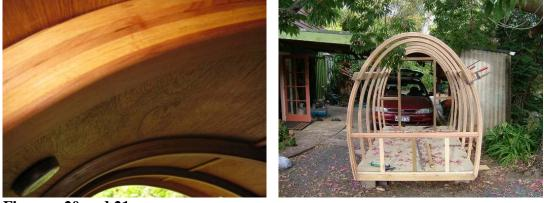
Figures: 20 and 21 Mark Astill finds totara sapwood bends and laminates well. It has also been used in boat-building for interior joinery.
