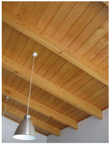
Figure: 62 Coloured-grade farm-totara sarking over macrocarpa rafters courtesy of John Guy.
