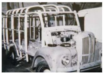
Silver beech timber was commonly used in vehicle framing for its combined strength and steam-bending properties.
