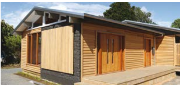
Managed stands of tōtara have the potential to become a significant regional timber resource. These offices in Kerikeri have weatherboards and joinery of milled farm tōtara.
